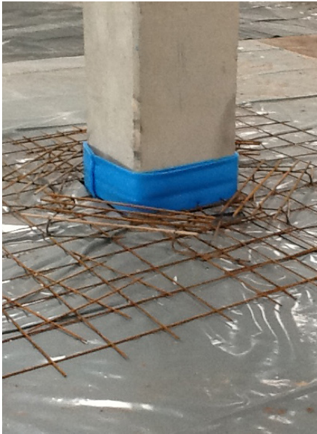
Structural insulation thickness - 5/10 mm
